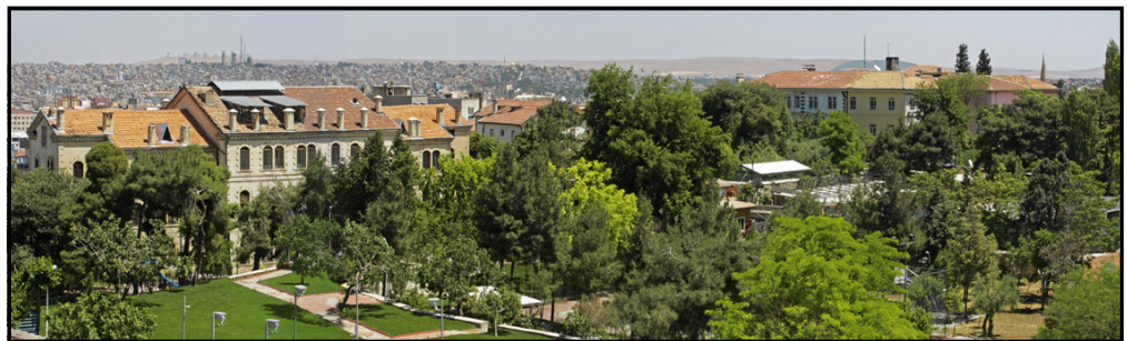
Panoramic view of the SEV American Hospital campus, Gaziantep
